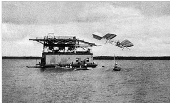
**Figure 2 Langley's Aerodrome during the test**
