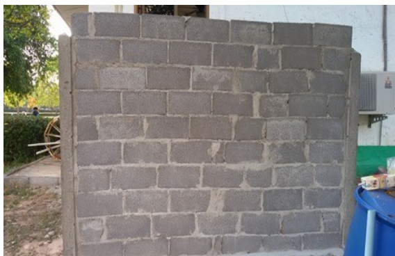
Figure 2 The concrete walls used in experimental preparation 2 x 2 meters.
