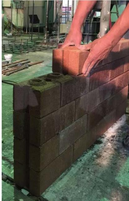
Figure 5 Typical construction of masonry walls
